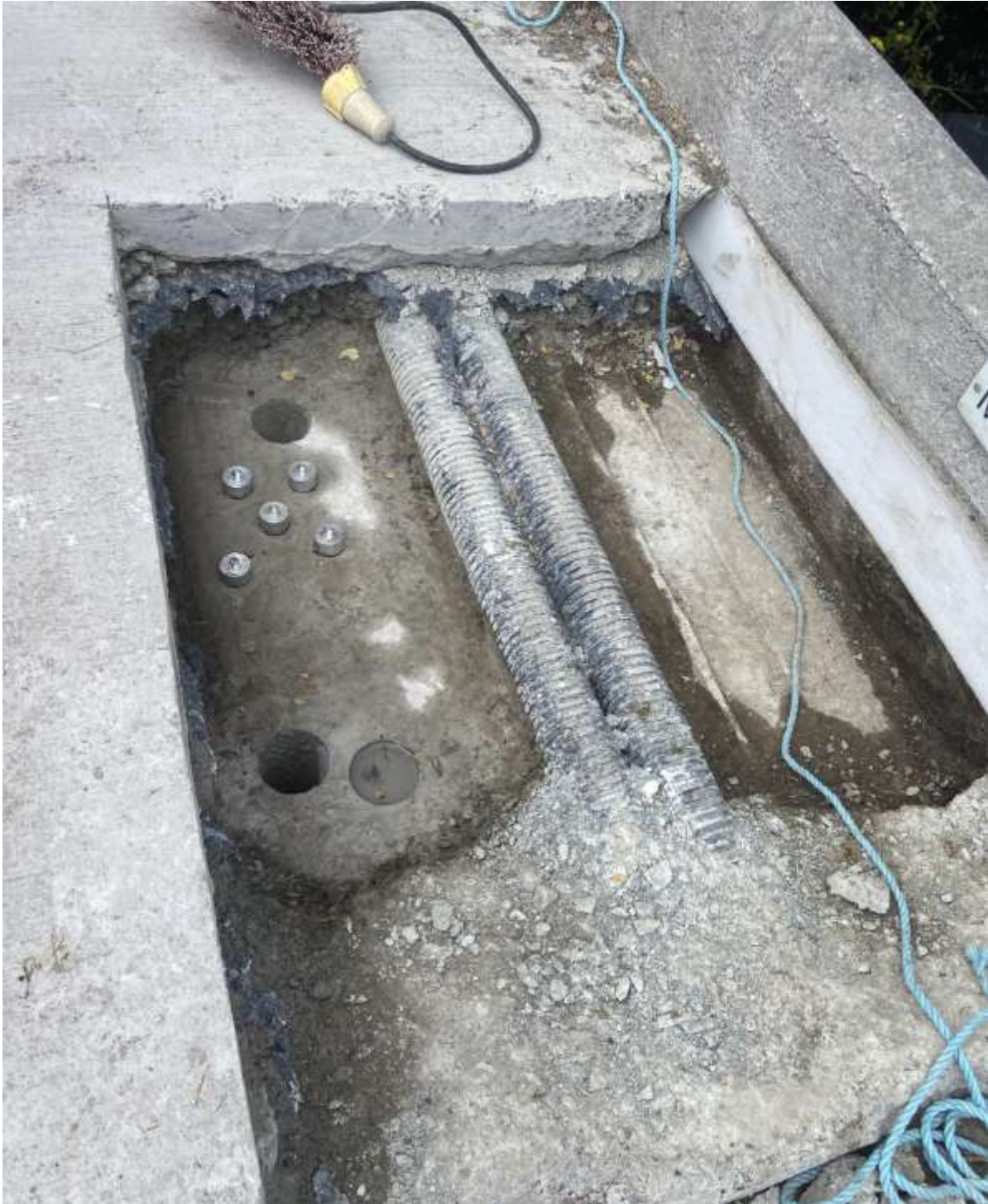
Figure 9: TA1 Cores 1,2 and adhesion test in place
