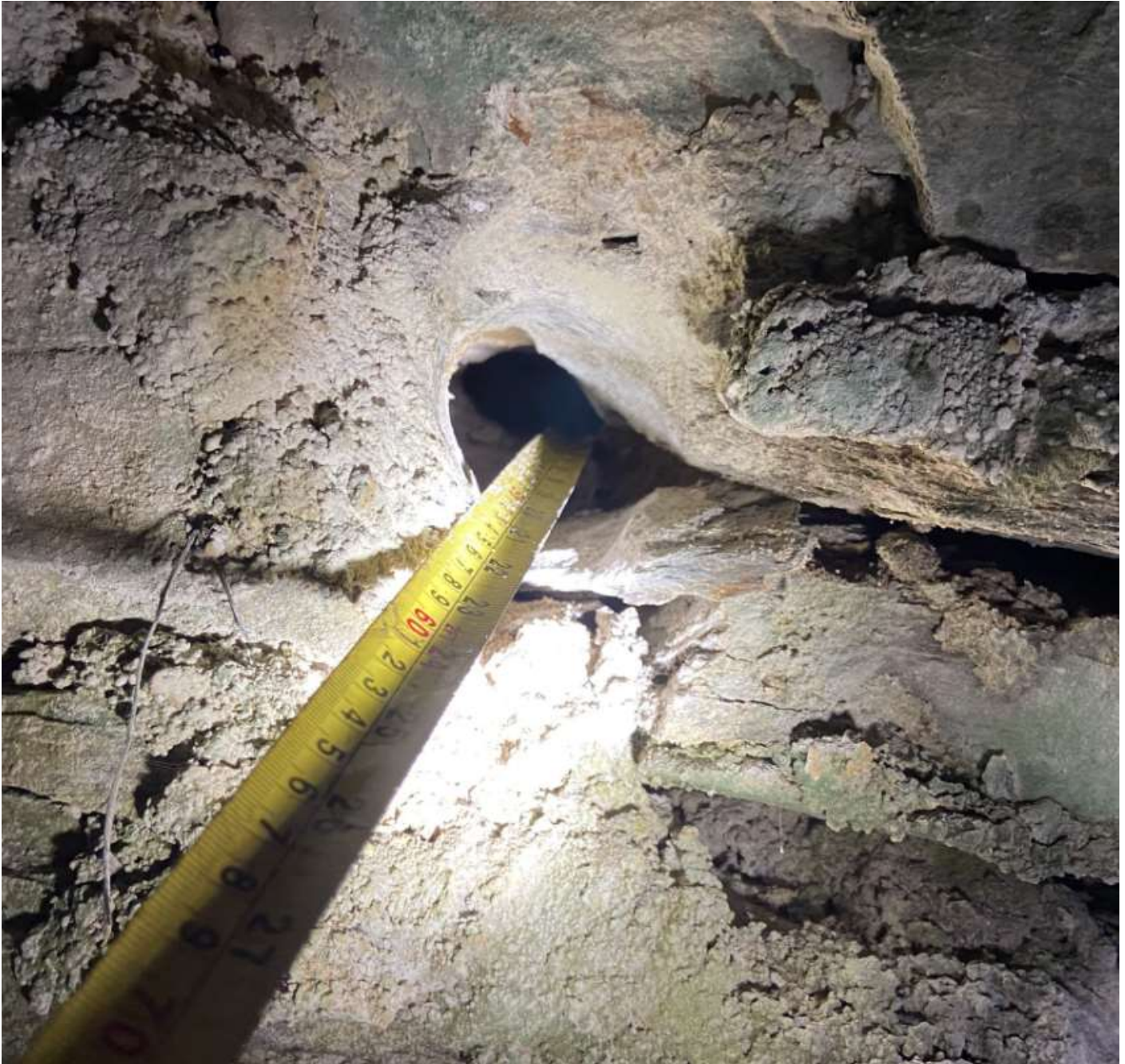
Figure 41: Pilot hole drilled through joint
