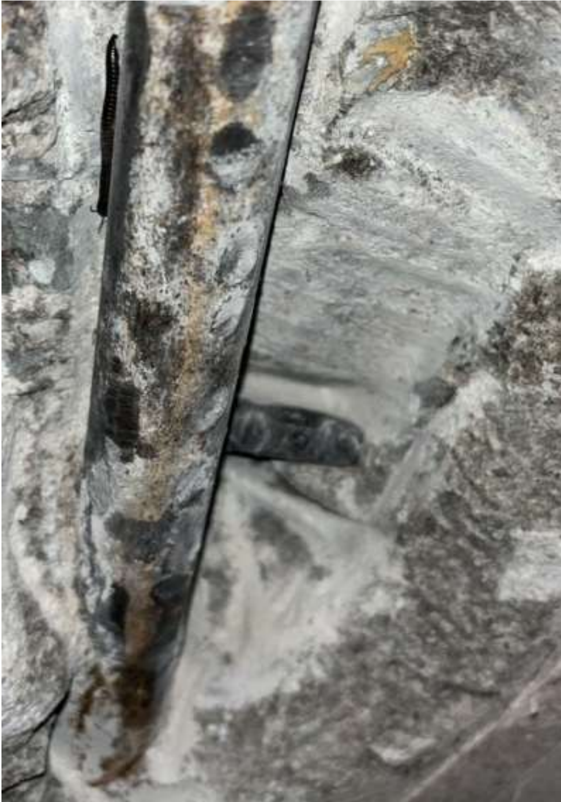
Figure 28: Transverse and Longitudinal smooth bar
