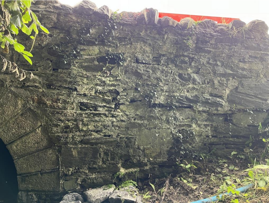
Photograph B-9 – View of the southeast wing wall
