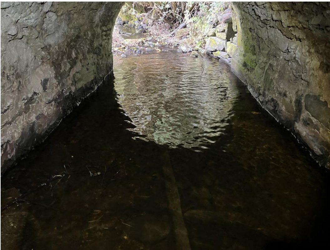
Photograph B-28 – View of the river at the south elevation of the structure
