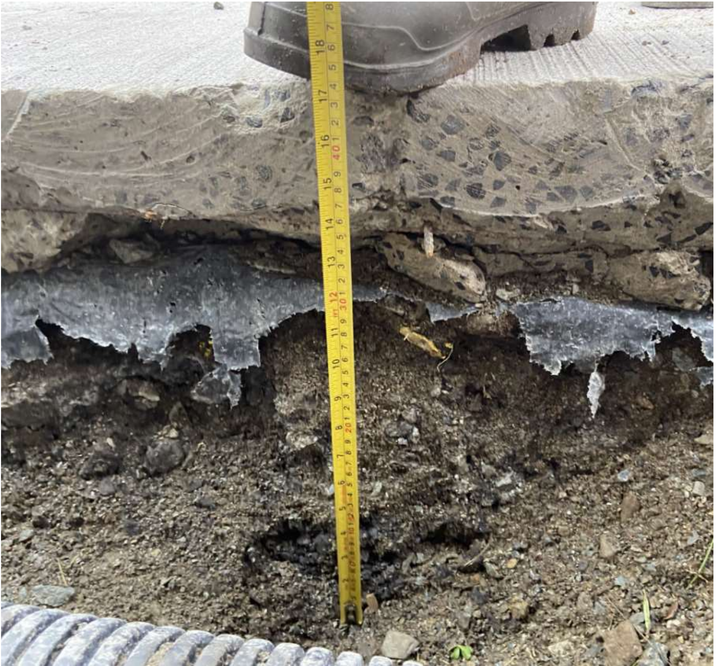
Figure 14: Fill layers above arch
