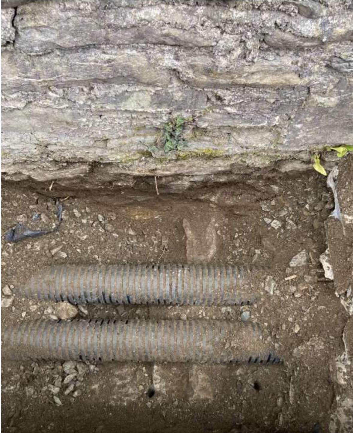
Figure 15: Pilot hole drilled through masonry in-line with keystone
