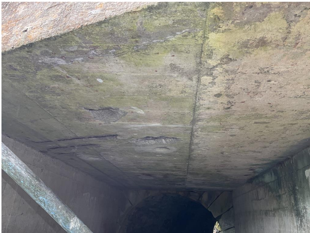
Photograph B-23 – View of the concrete deck extension looking south
