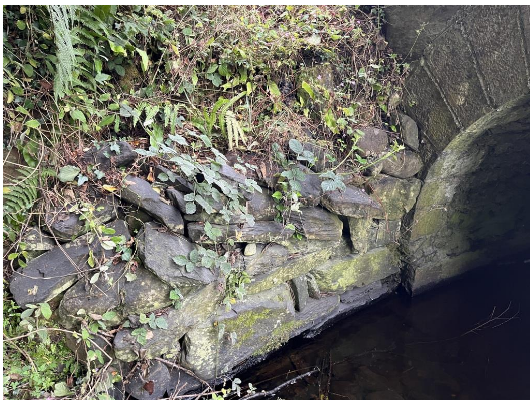
Photograph B-8 – View of the southwest embankment
