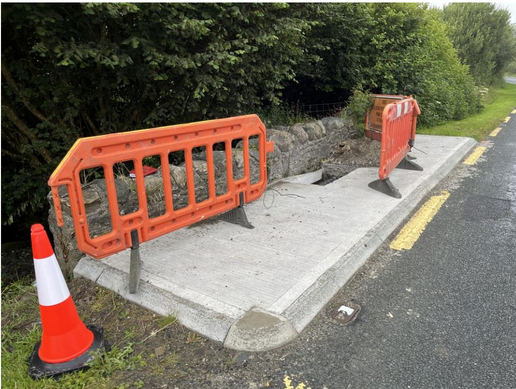
Photograph B-2 – View of the south rubbing strip and parapet
