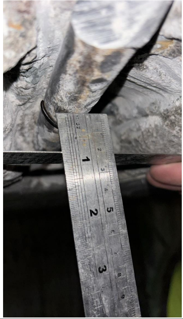
Area 4 smooth longitudinal rebar 22mm cover
