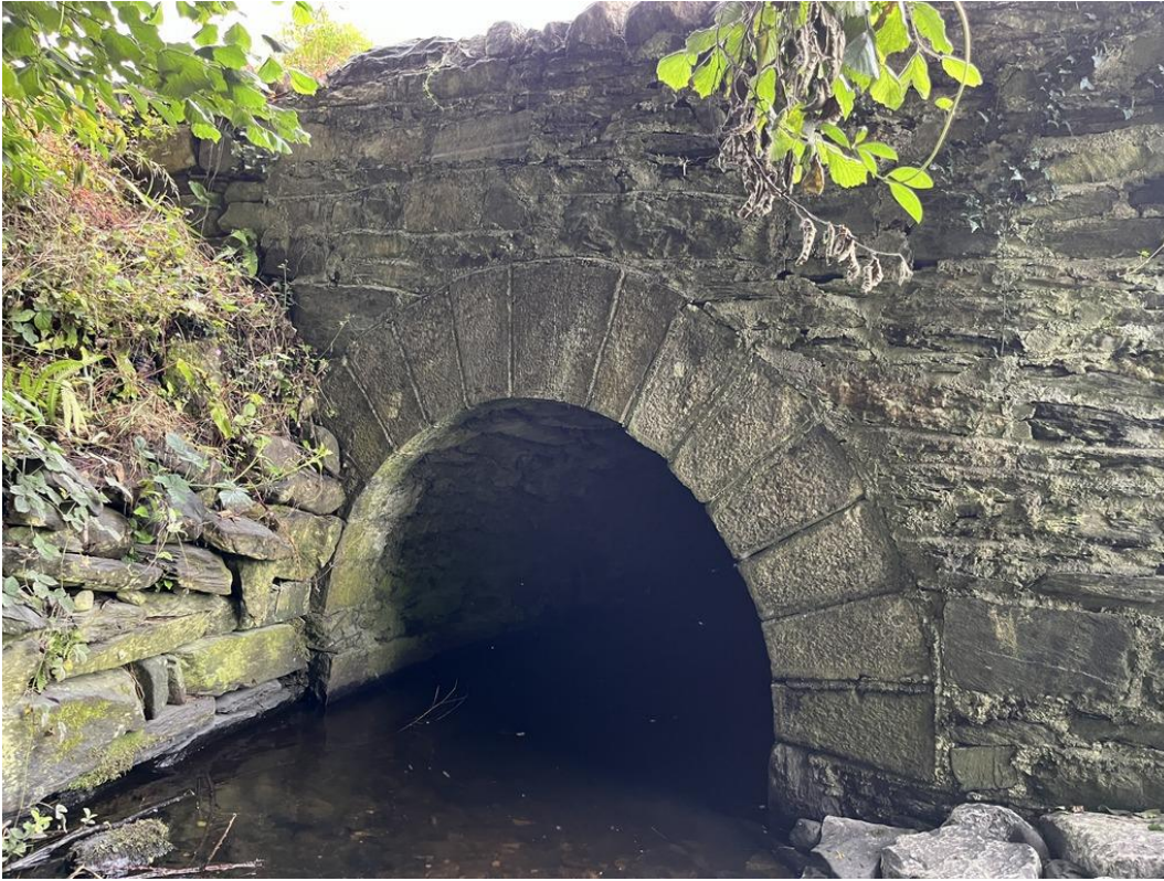
Photograph B-31 – View of the south elevation
