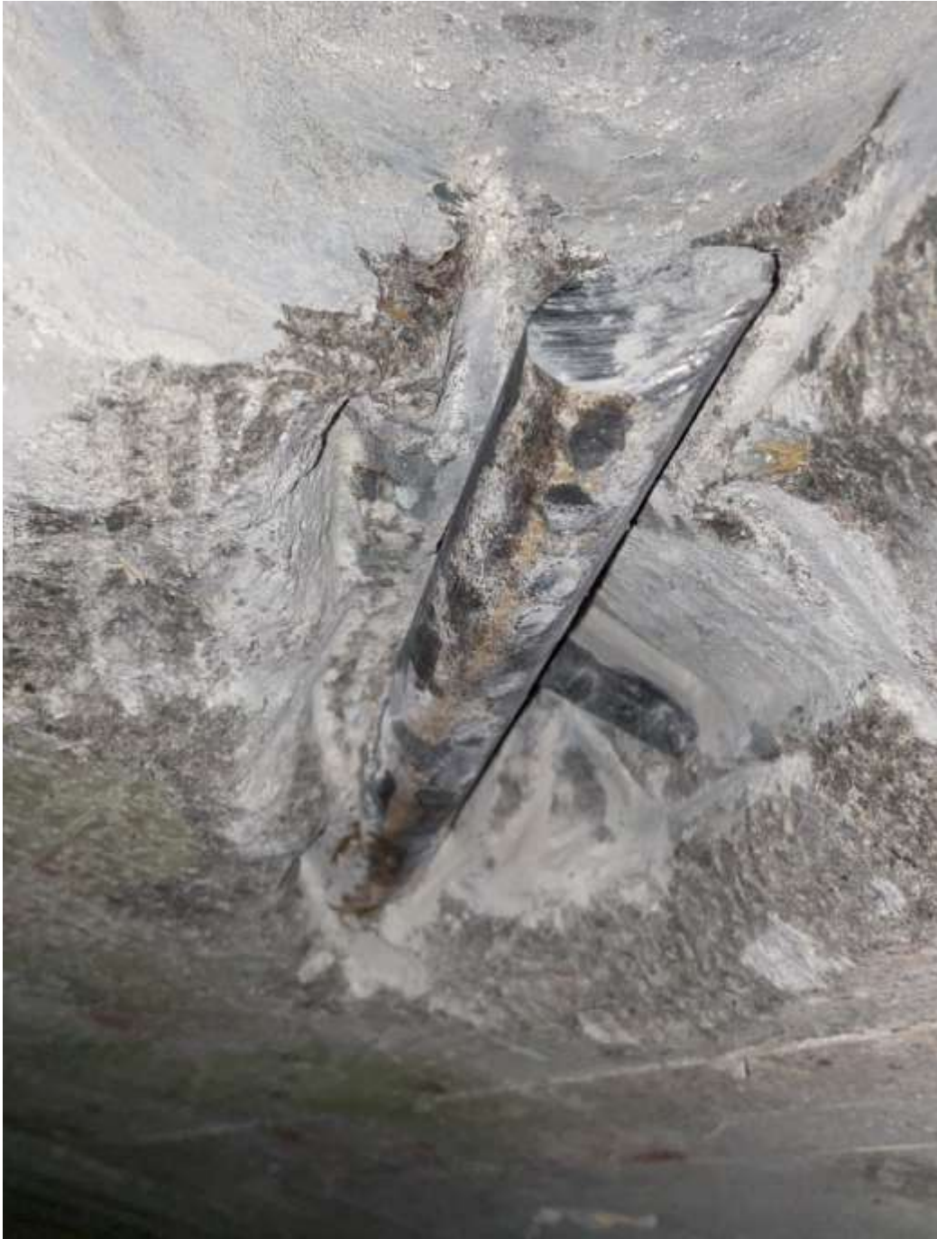
Figure 27 : Exposed Longitudinal and Transverse Reinforcement
