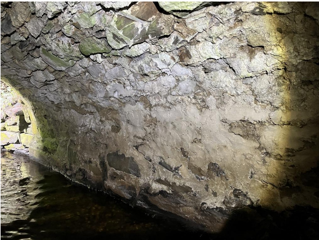
Photograph B-12 – View of the west masonry abutment
