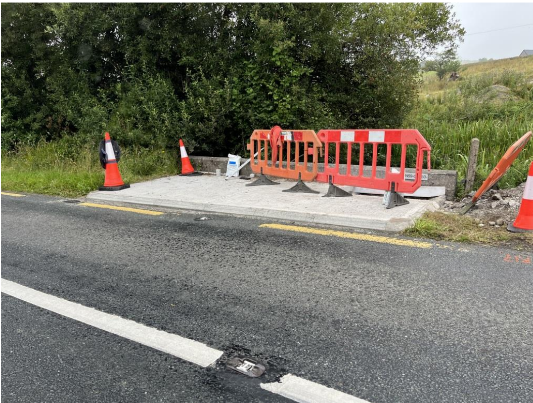
Photograph B-4 – View of the north concrete parapet
