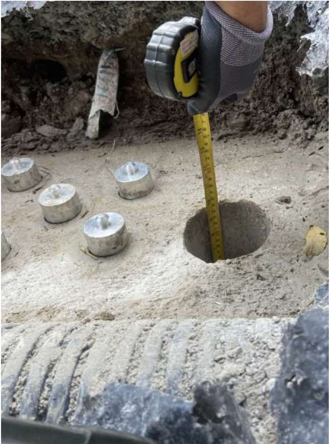
Figure 10: C1 /PH1 core hole depth measurement
