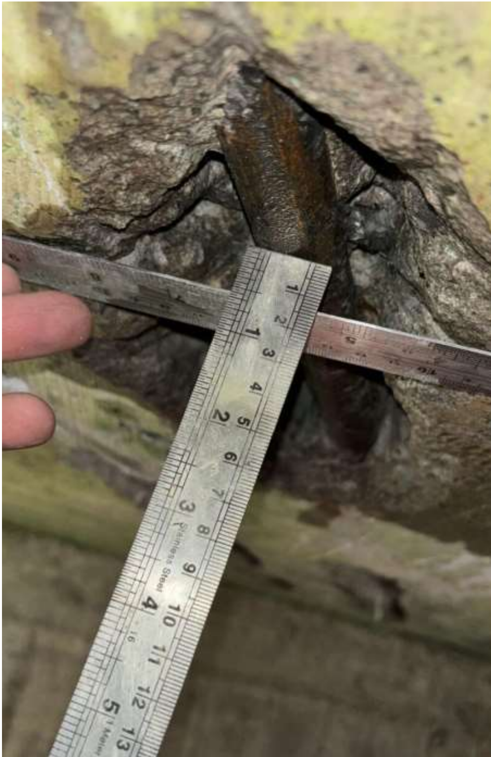
Figure 24: Measurement of cover
