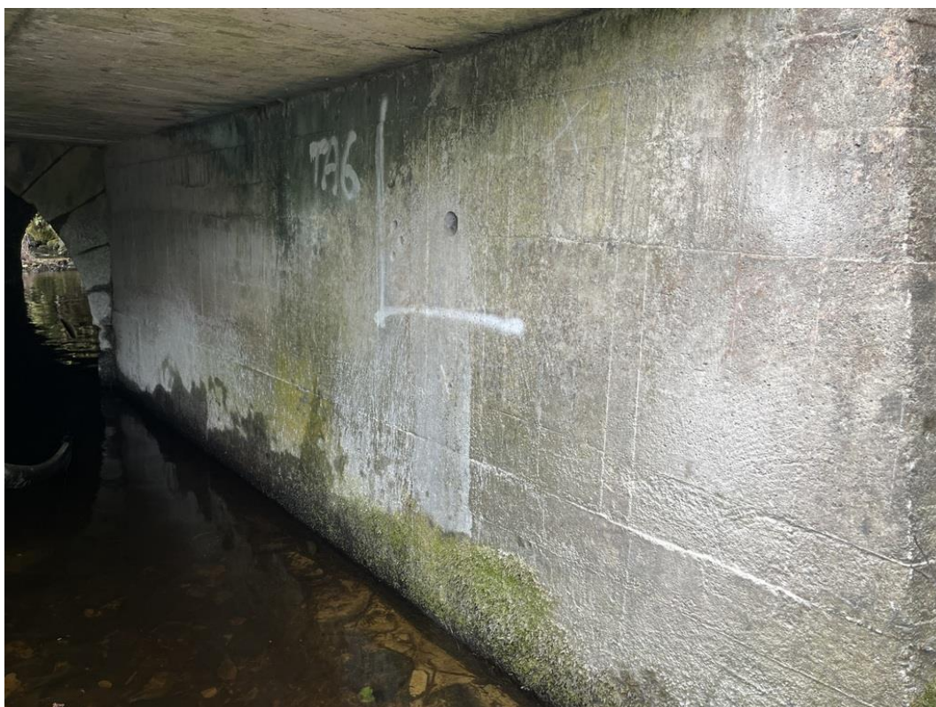
Photograph B-14 – View of the west concrete abutment
