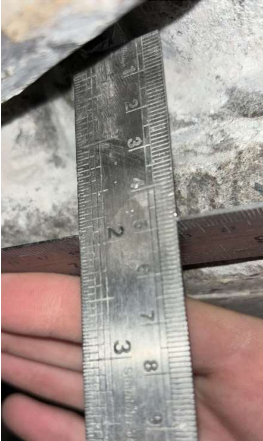
Figure 31: Cover measurement of reinforcement
