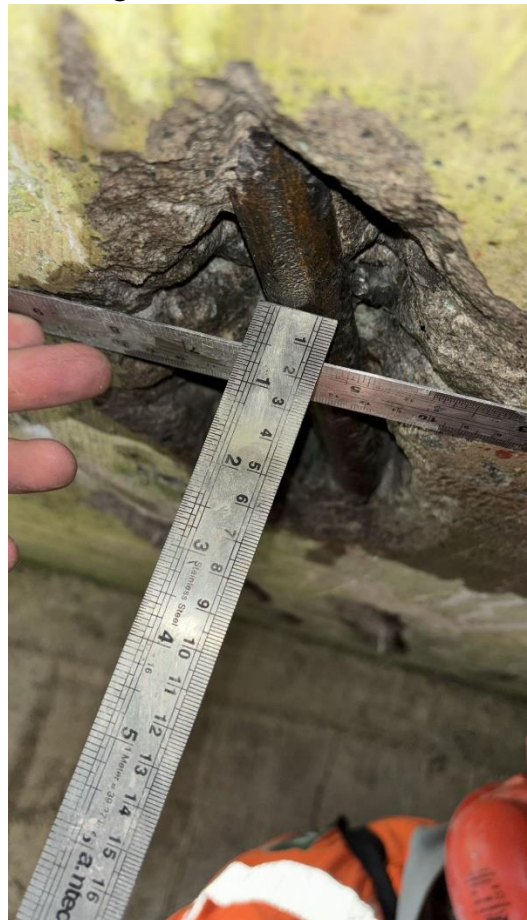
Area 3 Longitudinal smooth rebar 14mm cover
