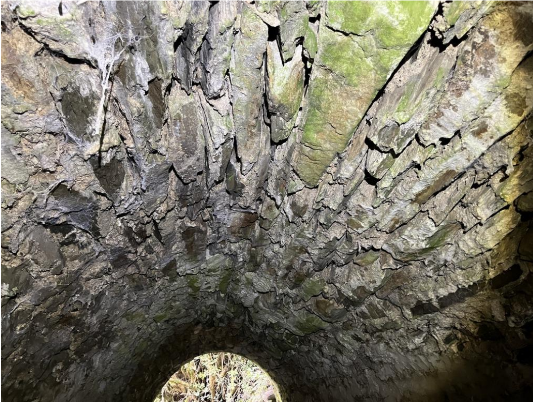
Photograph B-15 – View of the masonry arch barrel looking south
