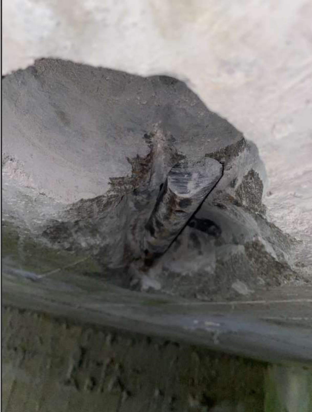
Figure 26: TA4 breakout area
