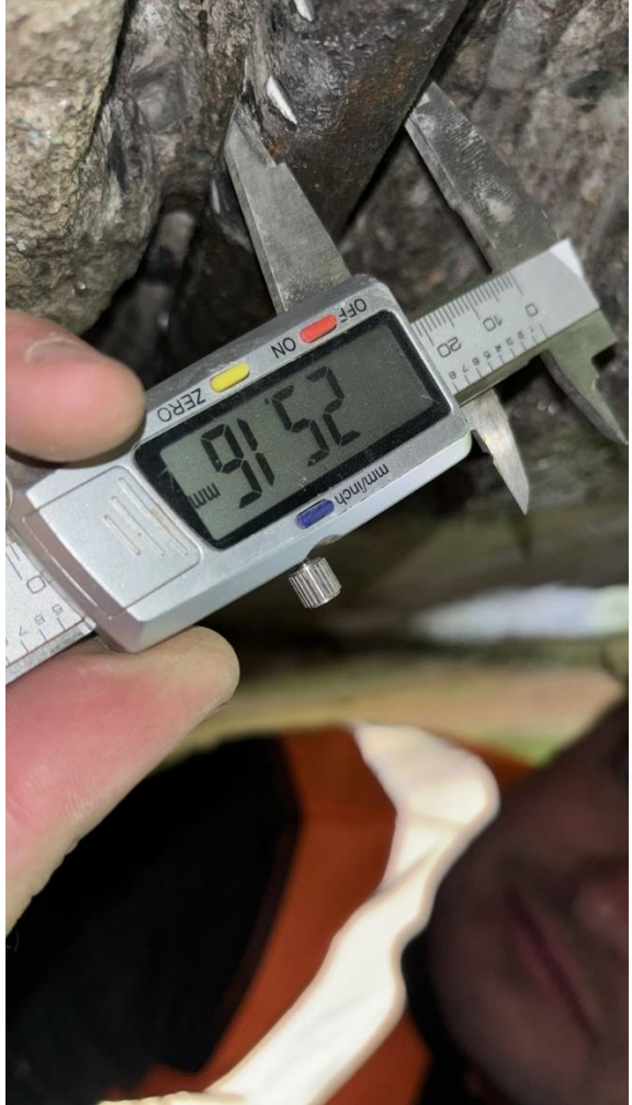
Area 3 Longitudinal smooth rebar 25.16mm
