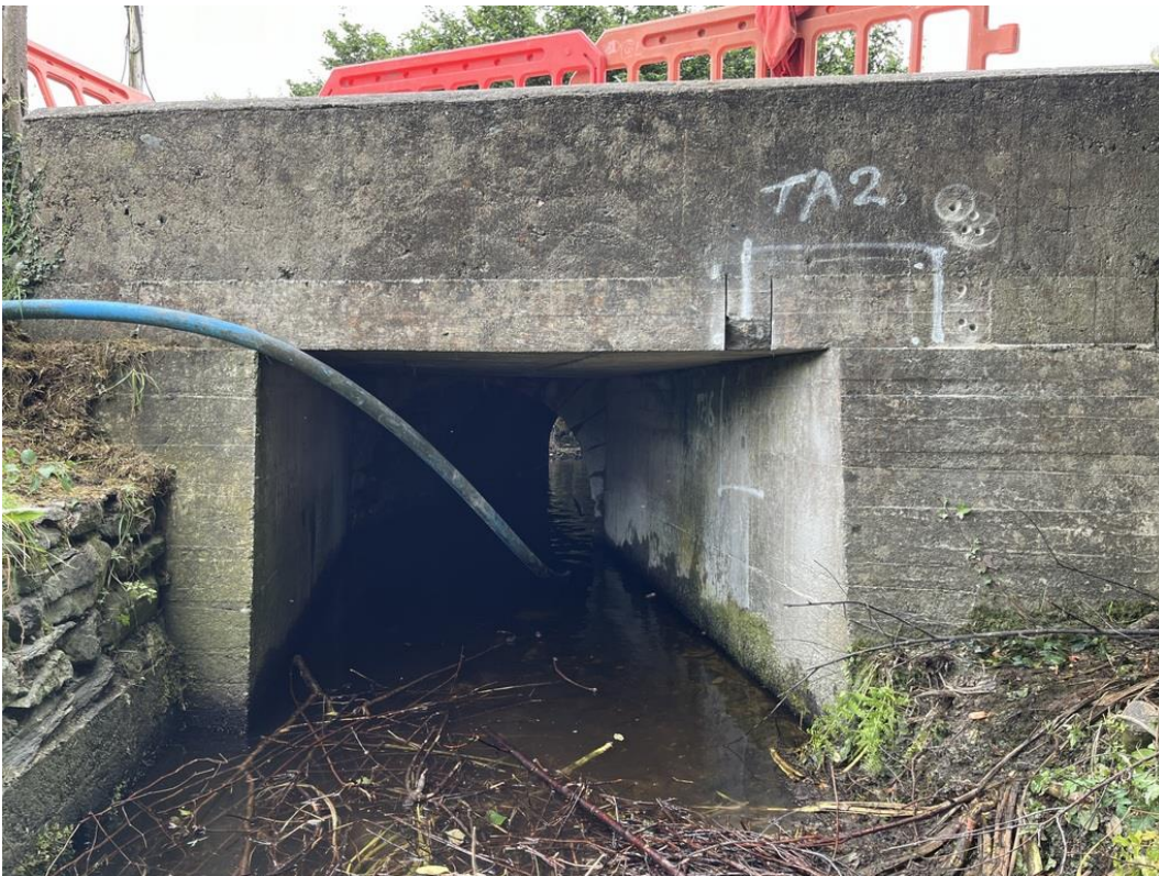
Photograph B-30 – View of the north elevation
