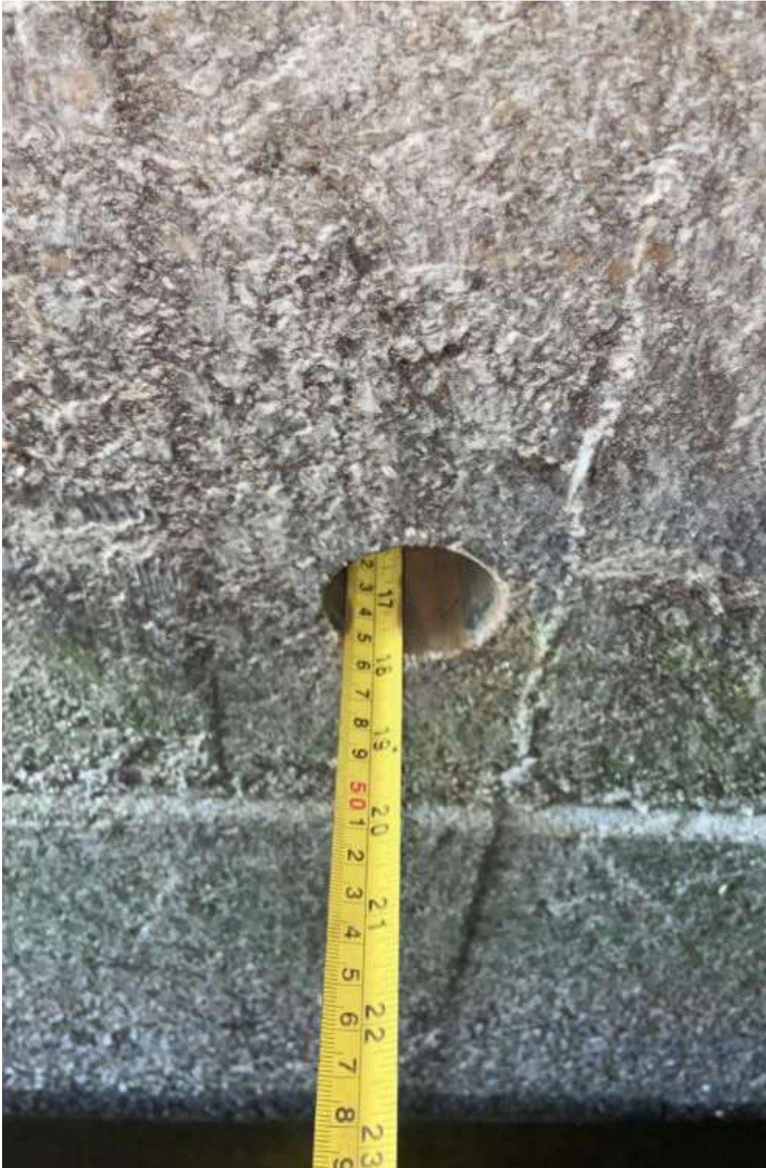
Figure 34: Pilot hole depth measurement
