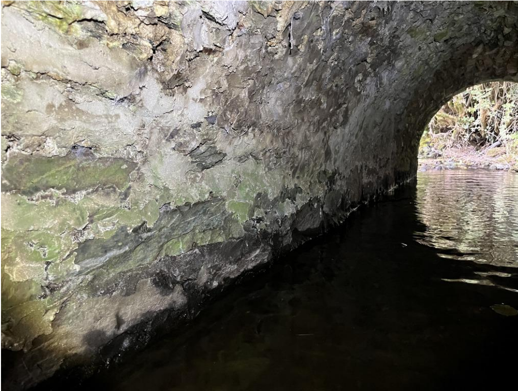
Photograph B-11 – View of the east masonry abutment
