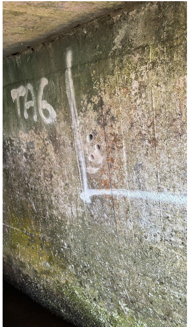
Area 6 West Abutment
