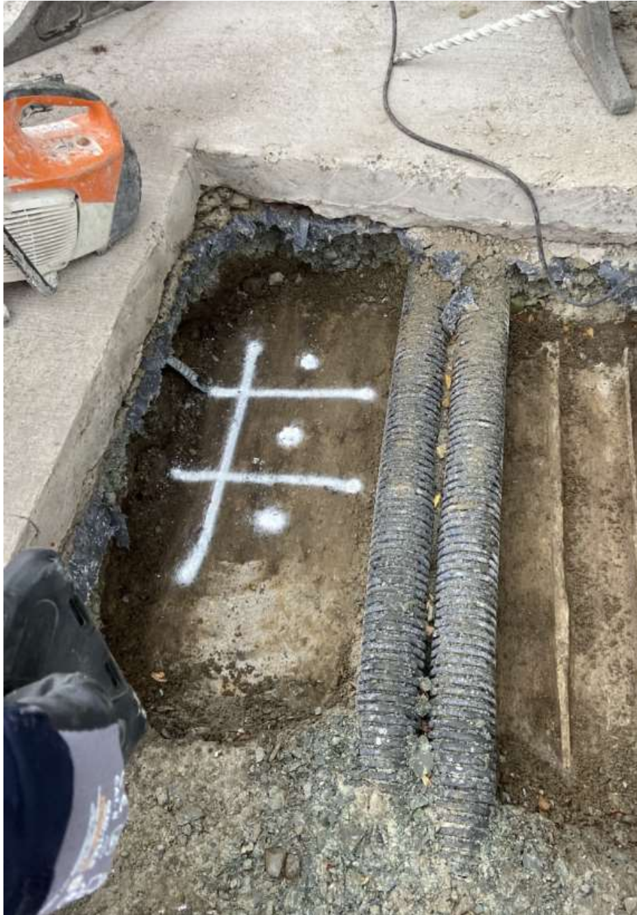
Figure 8: Deck scan of reinforcement( located on soffit side)
