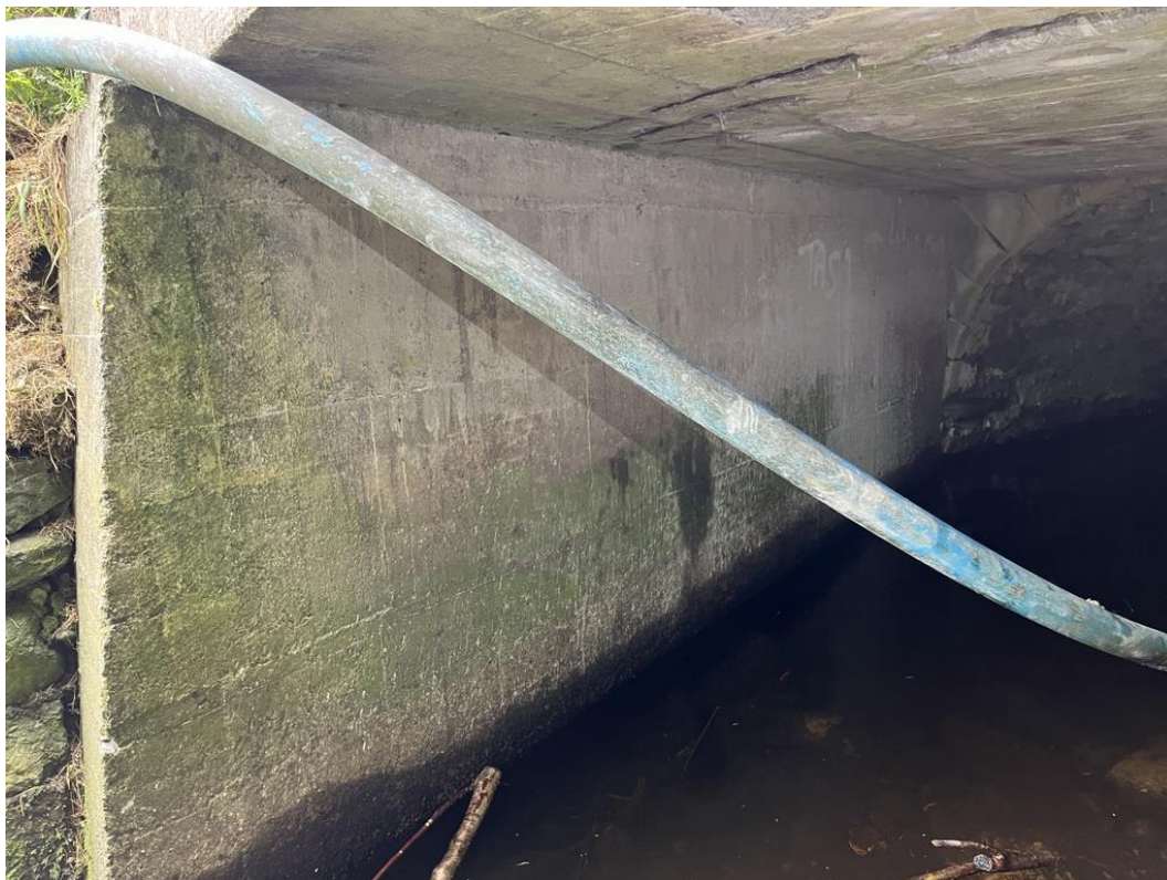
Photograph B-13 – View of the east concrete abutment
