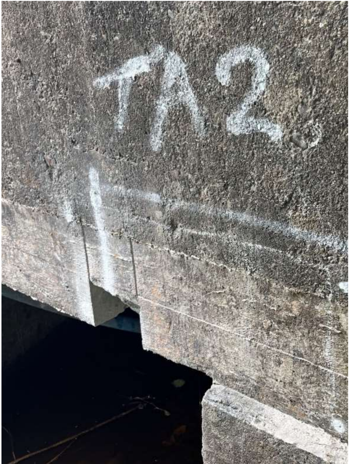
Figure 17: Test area 2 breakout
