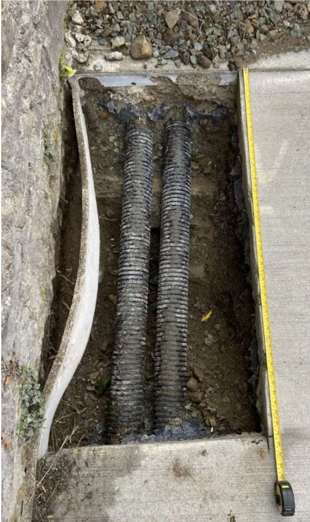
Figure 13: Ducts exposed above arch
