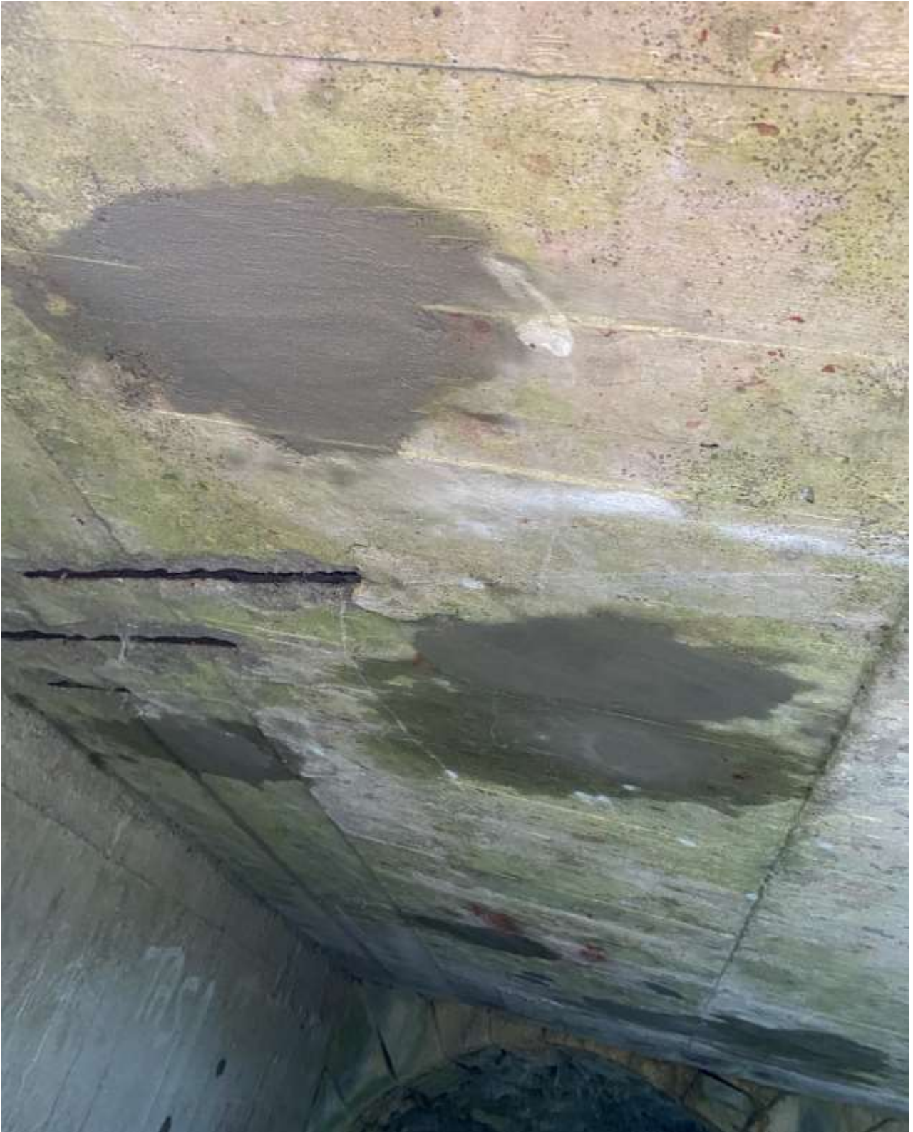
Figure 25:TA3 and TA4 reinstatement
