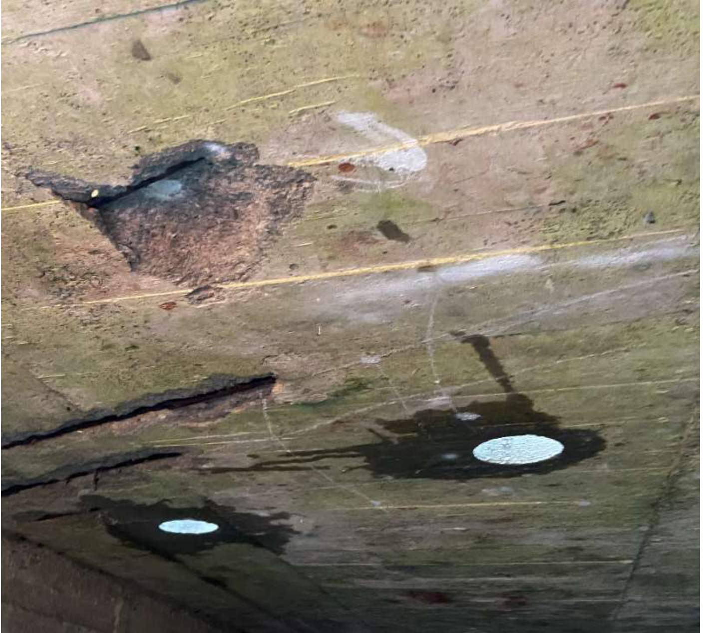
Figure 20: TA3 scanned area (Reinforcement marked with white chalk)
