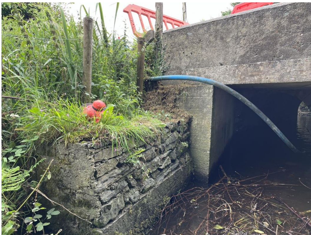
Photograph B-7 – View of the northeast embankment
