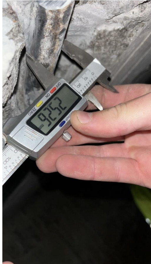
Area 4 Longitudinal smooth rebar 25.26mm
