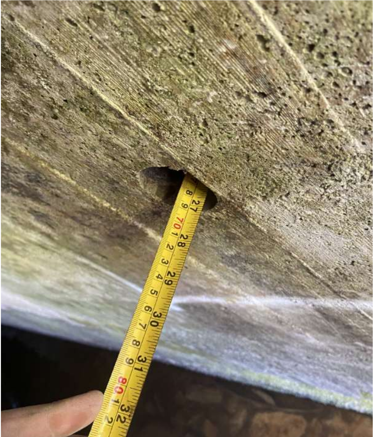
Figure 38: Pilot hole depth measurement
