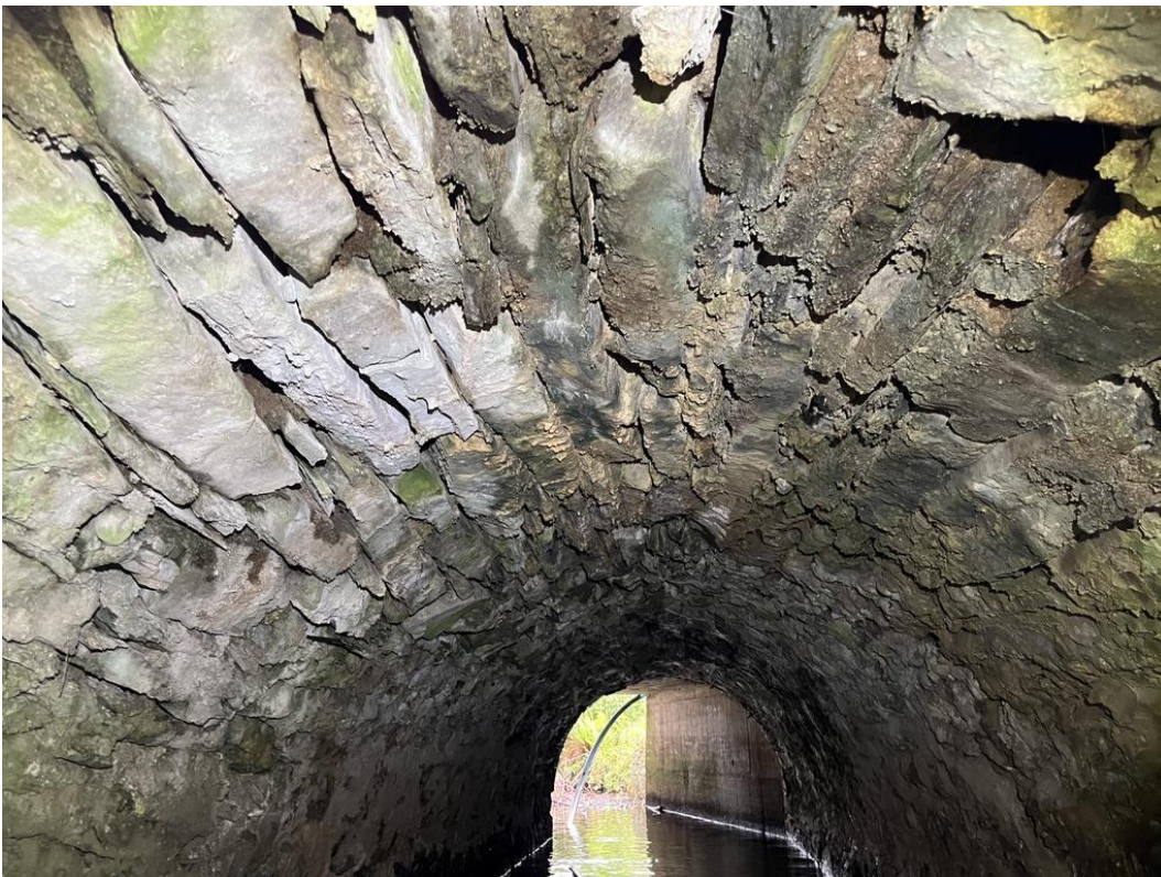
Photograph B-16 – View of the masonry arch barrel looking north
