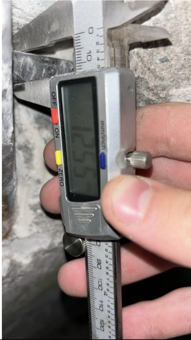
Area 4 transverse smooth rebar 12.55mm
