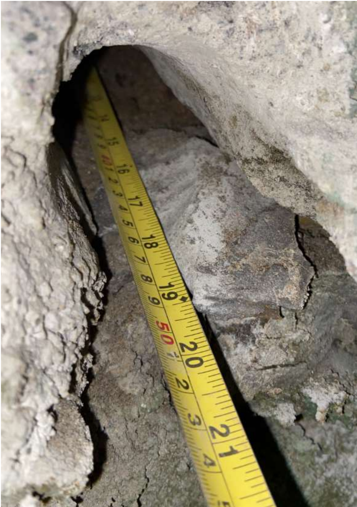
Figure 43: Measurement of pilot hole depth
